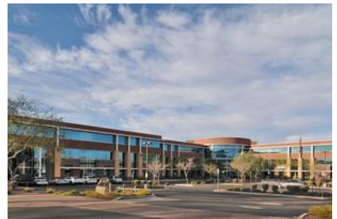
Oaktree Capital bought buildings III and IV at the Raintree Corporate Center in Scottsdale.
